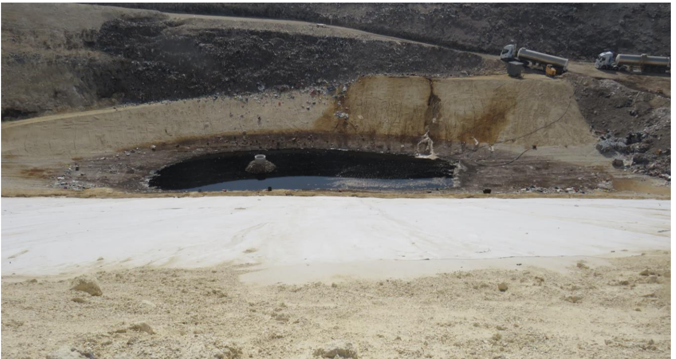
Photo 2: Leachate pool at the bottom of Cell 9
